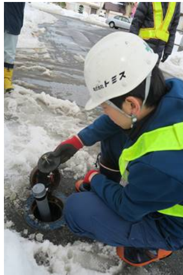
Installing a transmitter in a manhole
