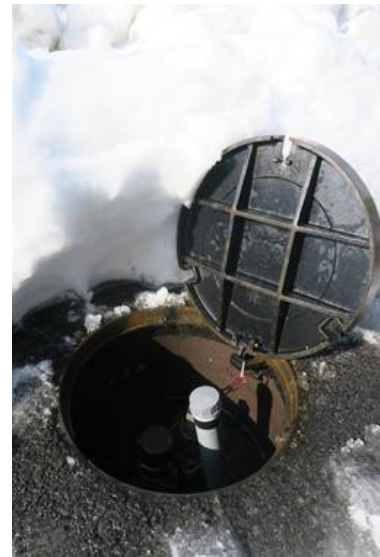
Installing a transmitter in a manhole
