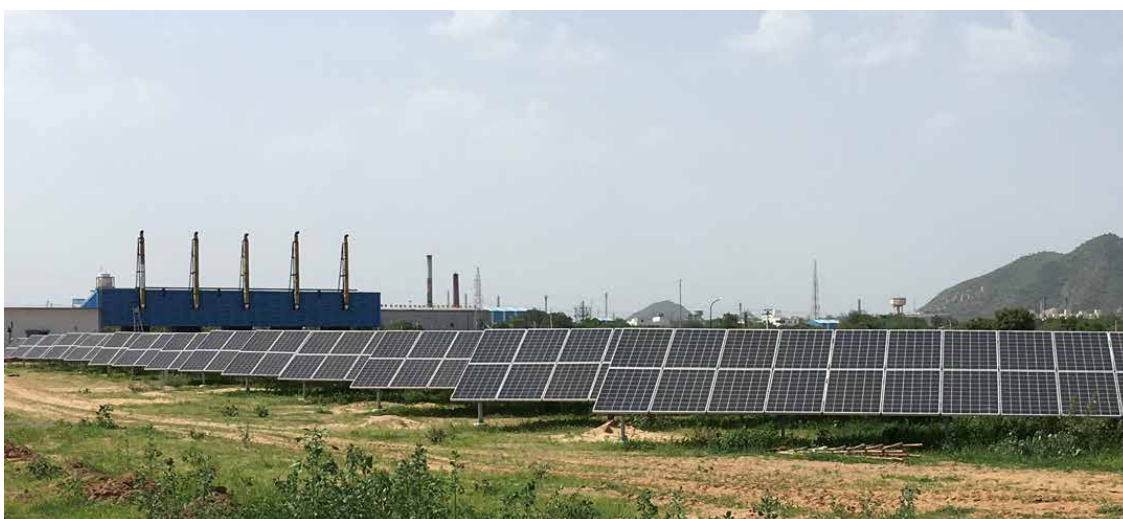
Figure 1. Microgrid system using PV power generation
